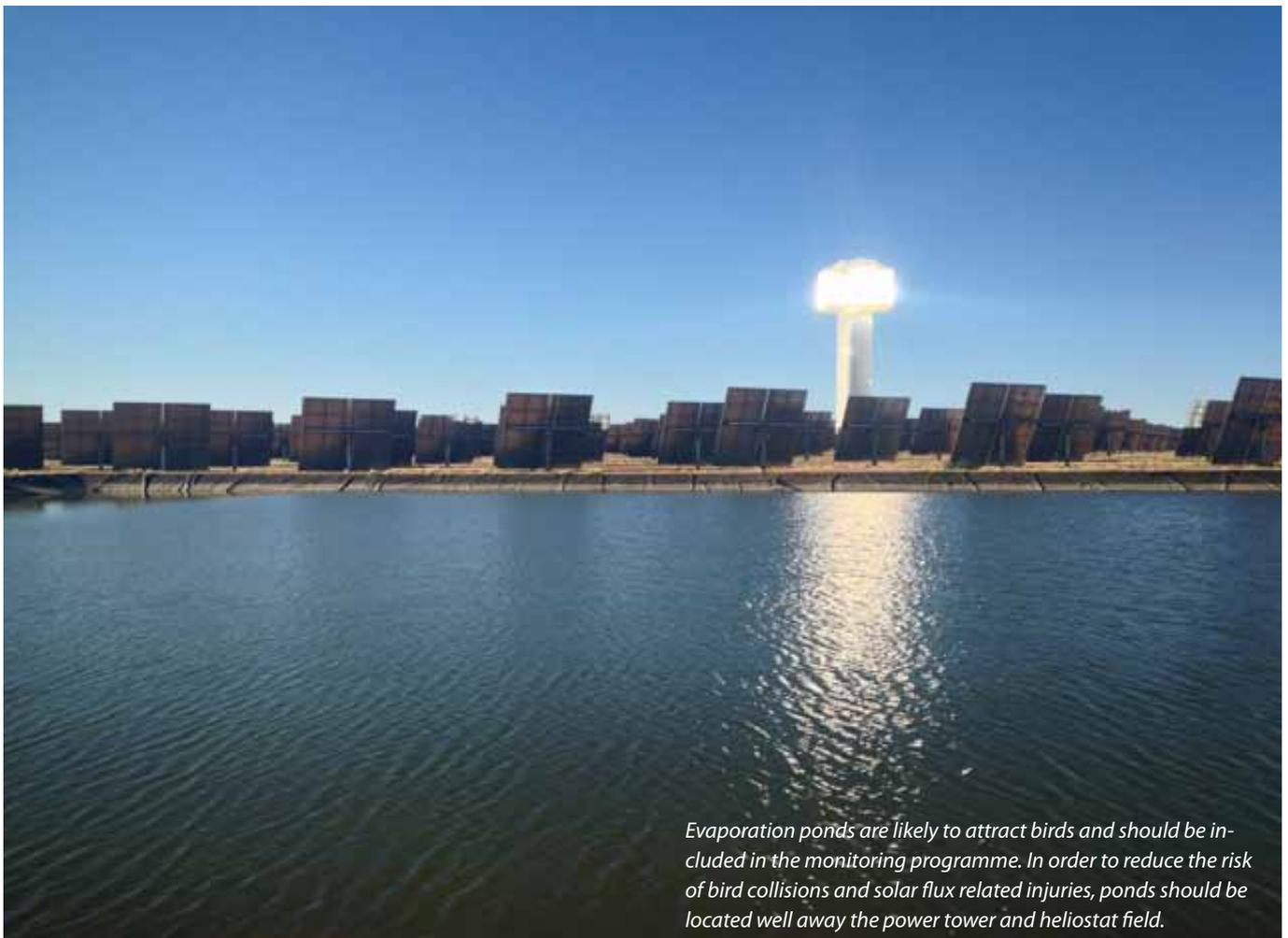
*Evaporation ponds are likely to attract birds and should be included in the monitoring programme. In order to reduce the risk of bird collisions and solar flux related injuries, ponds should be located well away the power tower and heliostat field.*
