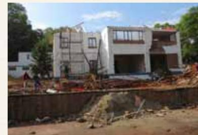
*The roof had to be replaced, but the shell of the building was reused.*
